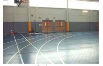
south wall entrance doors
