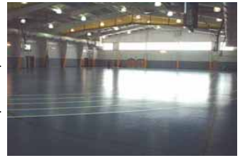
north west corner looking towards south wall
