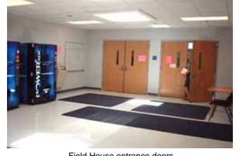
Field House entrance doors
