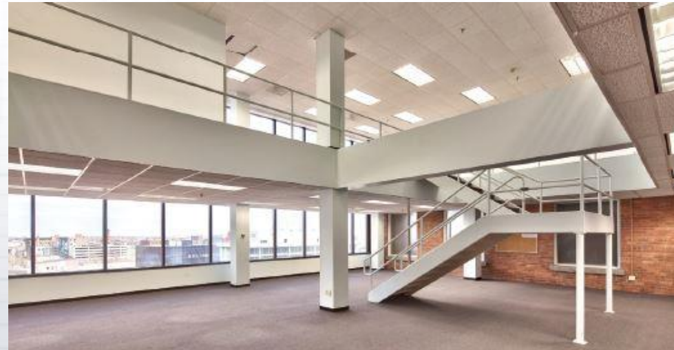
Ellwanger and Barry Building, 39 State St
